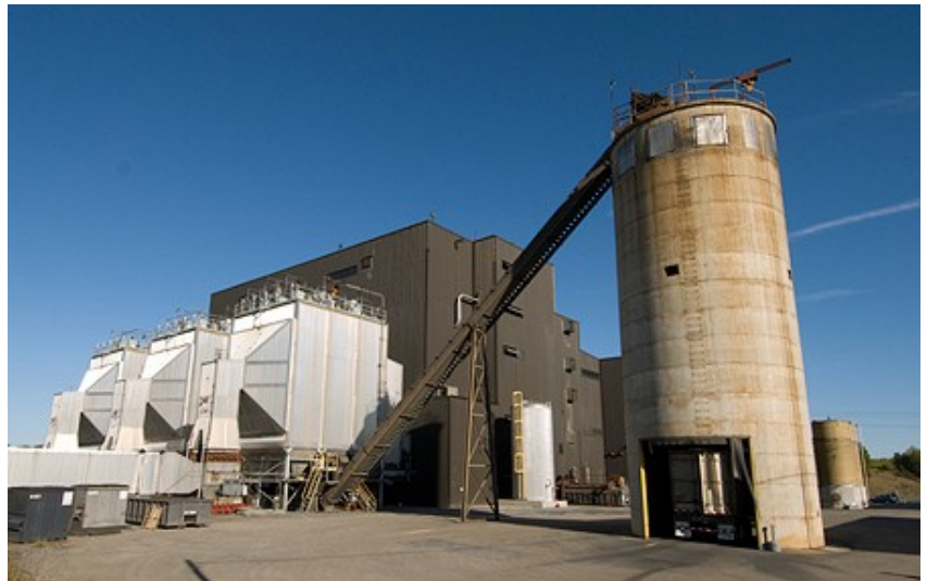
Dominion's Hurt Power Plant in Pittsylvania County
